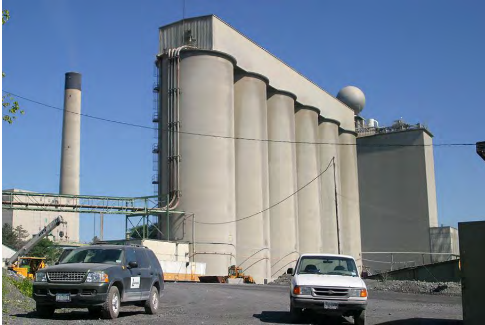
Figure 8: Ball reservoir located on top of Pack-house.
